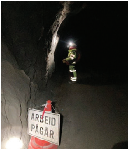
Geological mapping of underground tunnel (there is no light besides torches)
